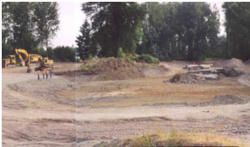
Butte Pit During Construction
