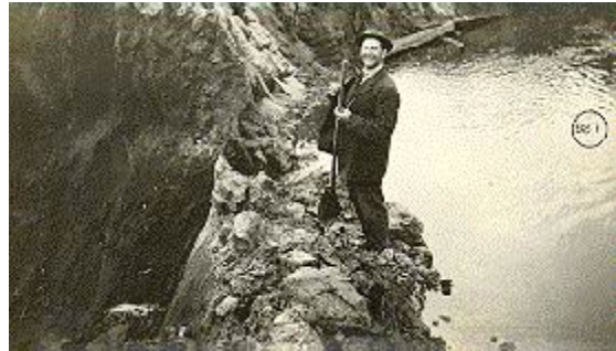
Brush mats were woven on a catamaran and set in place with rocks for bank stabilization. May 1916
