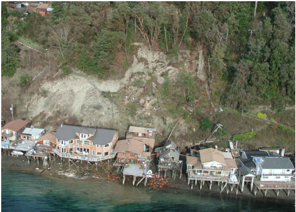
Figure 4.G2-2 Salmon Beach, Tacoma Washington – Following Feb. 2001 Earthquake
