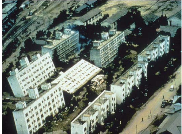
Figure 4.G2-2 Liquefaction, Niigata Japan 1964
