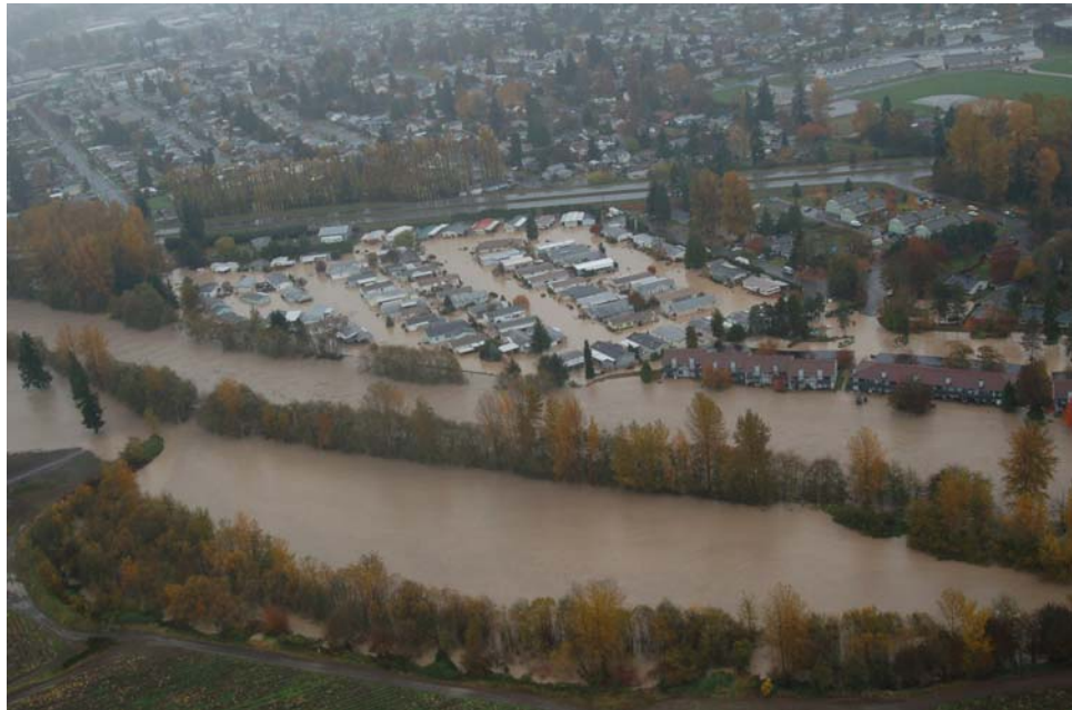
Figure 4.M3-4 Nov. 2006 Flooding Rainier Manor – Along Puyallup River
