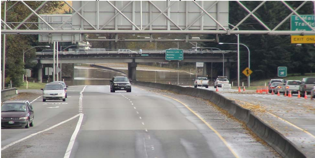
Figure 4.M3-3 Nov. 2006 Flooding State Route 410 – Along Puyallup River
