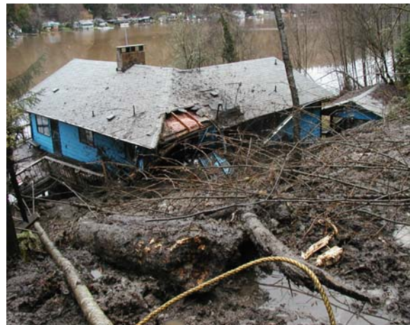
Figure 4.G3-2 Ski Park Road – Landslide 01/31/03
