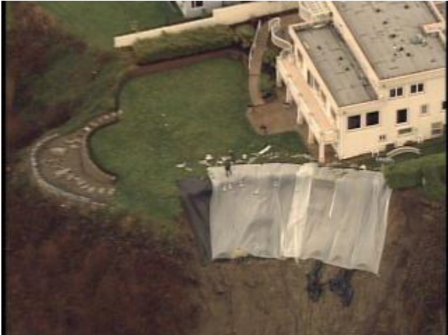
Figure 4.G3-1 Northeast Tacoma – Landslide 01/2007
