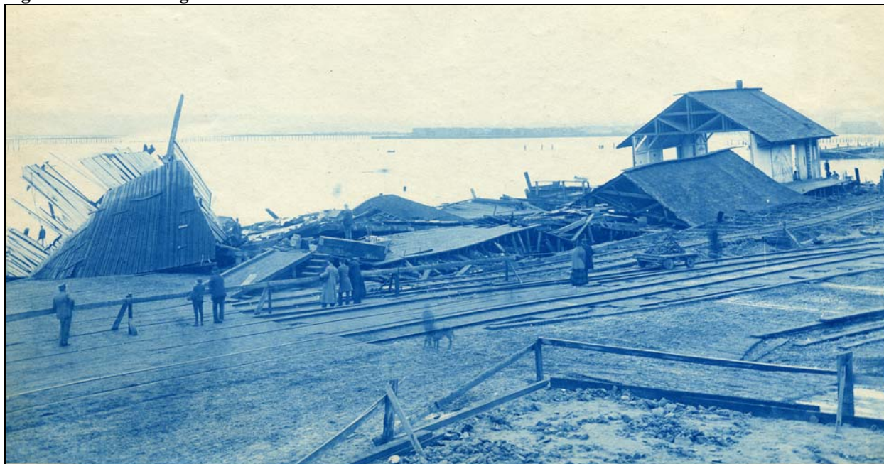
Figure 4.G4-11 Damage in Tacoma from the 1894 Tsunami 21
