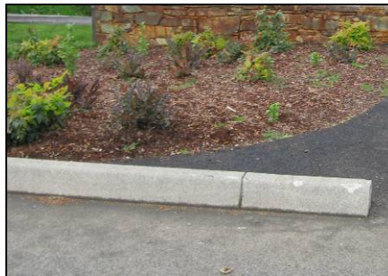
Existing curb stop
