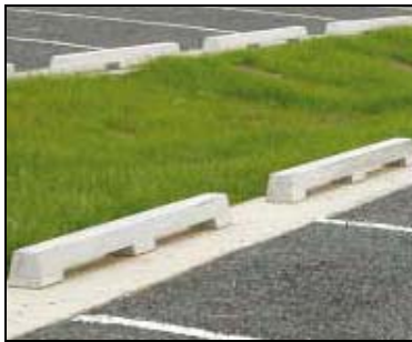
Open curb stop
