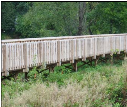
Tualatin Greenway Pin-pile boardwalk
