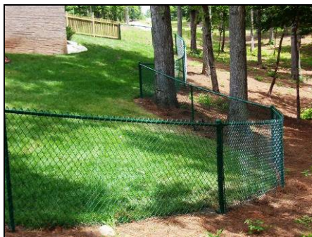
Green coated chain-link fencing
