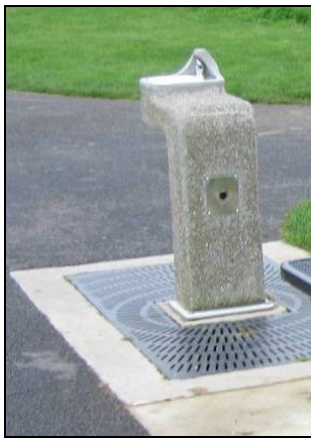
Existing water fountain
