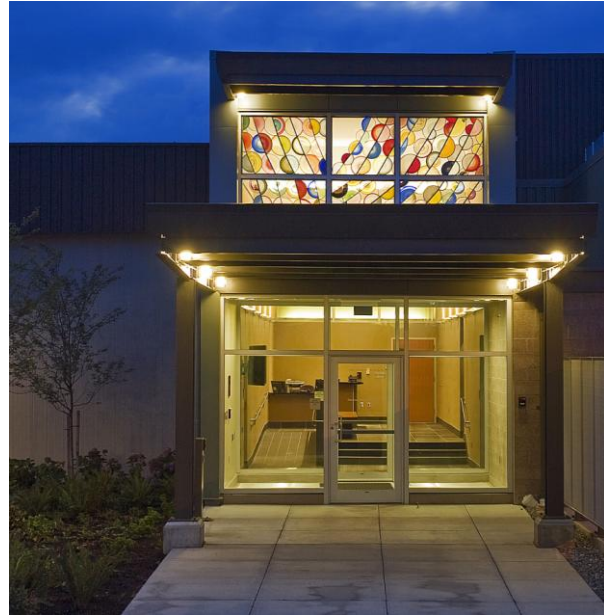
Reemergence, 2008 by Benjamin Moore and Dick Weiss Hand-blown and leaded glass window, six panels Emergency Operations Center, Tacoma Pierce County 1% for Art Program
