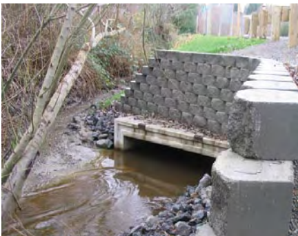
The Artondale culvert, completed in 2004, stabilizes the roadway and helps drainage.
