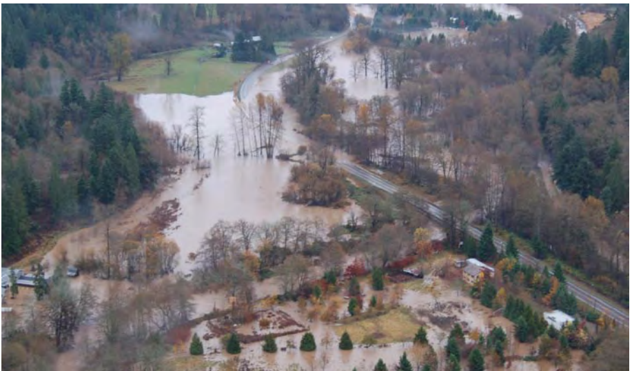
South Prairie Creek floods across State Route 162, November 2006.
