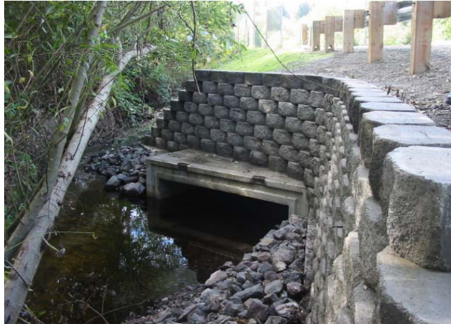
A capital improvement project
