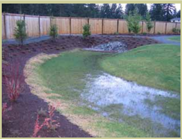
Stormwater drainage bioswale with level spreader, Frederickson. Jan 2006.
