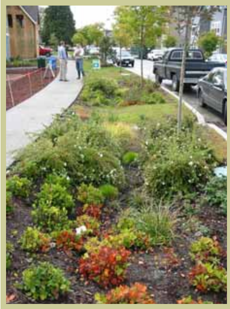
Drainage bioswale planted with native plant species, High Point Neighborhood, Seattle. Sept 2006.
