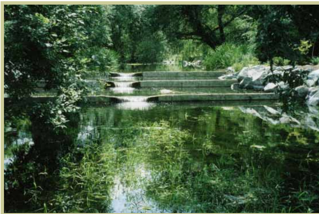
Fish ladder on Clover Creek, Lakewood.
